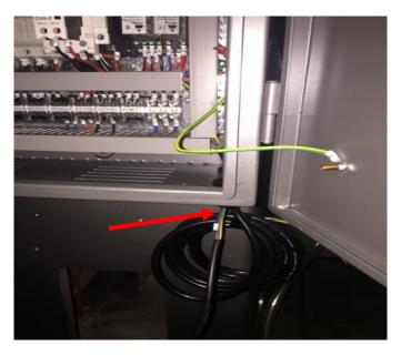
6. Connect the pump wires to U1 & W1 in terminal plate. If the pump does not run, change the U1 to V1 position which is power source wire.
