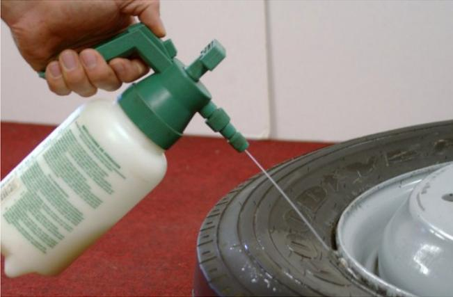
**Generously lubricate both sides of the tire before demounting. NOTE: We recommend using liquid lubricant to penetrate between rim and tire bead for demounting.**
