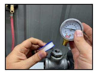
3. Locate the output hose gauge. Pipe Tape or Pipe thread will help with indexing the gauge for ease of use.
